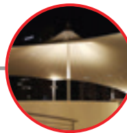
Fabric Shade Structure
