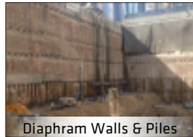
Diaphragm Walls & Piles
