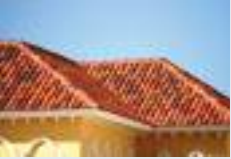
Clay Tile Roofing
