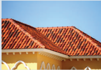
Clay Tile Roofing
