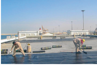
ROOFING AND WATERPROOFING
