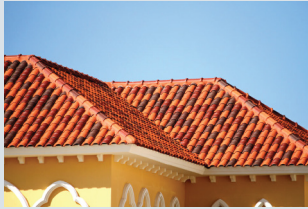
CLAY TILE ROOFING
