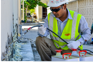
CRACK INJECTION
