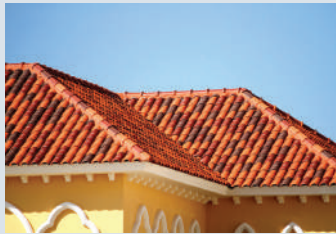
Clay Tile Roofing
