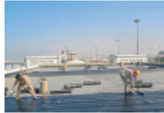
Roof Waterproofing
